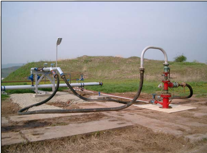
Above; Drill crew getting ready. Below; A typical solution mine well head and distributor.
