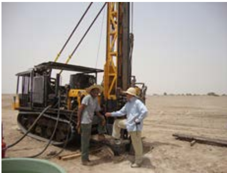
Exploration Drill Rig
