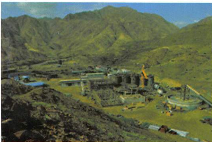
Fig 3 – Process Plant under construction
