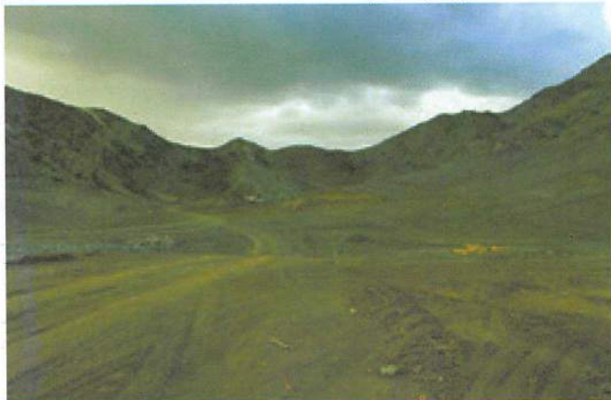
Fig 8 - TSF Basin Preparation
